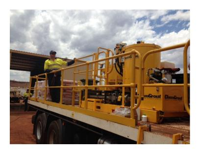
Shortly after being mixed, the bentonite is pumped through an in-line grout pressure gauge passing through a Tremie line to the desired depth. Over 37 cubic metres of bentonite was batched and pumped over the first stage. The highly efficient colloidal mixer makes possible water to cement ratios down to 0.35 by weight, resulting in very high strength grouts with little if any bleed water release.
