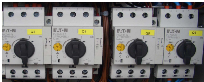
Fig. 1: Motor protection switch
